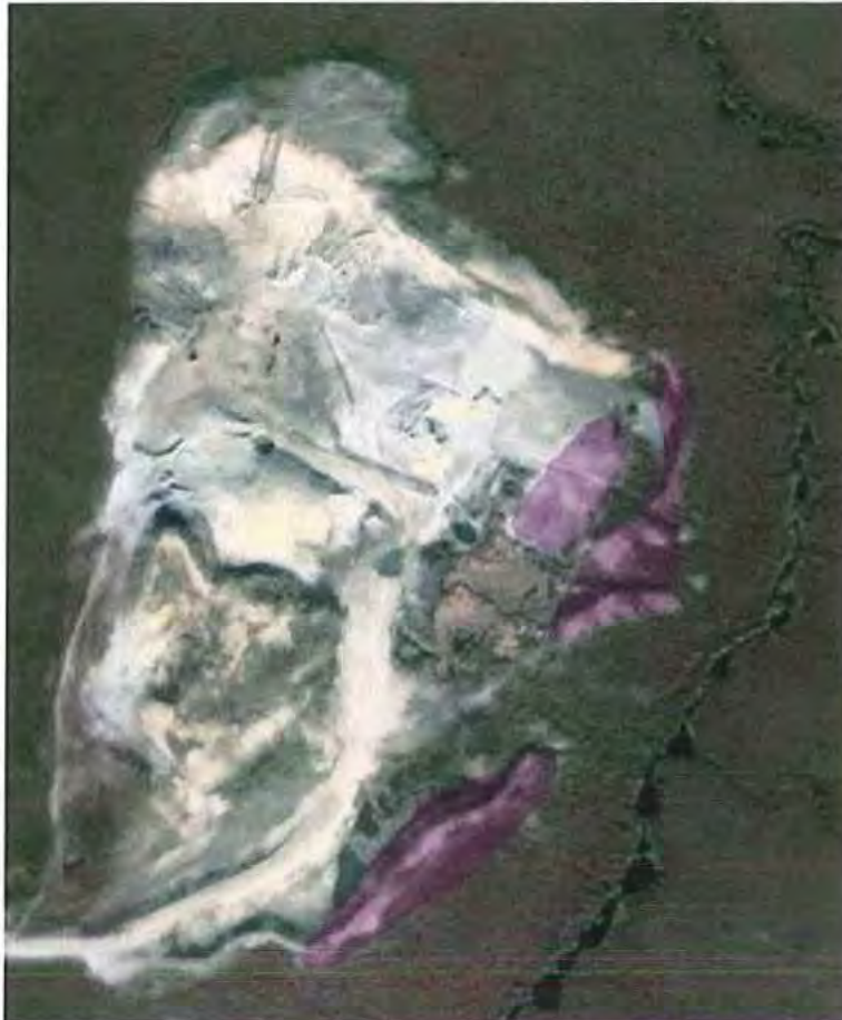
Photo 1: Google Earth ® Aerial View of Hotham Peak Quarry (5/30/2012). Proposed reclamation areas (shaded purple) approximate, since the imagery is not current.
